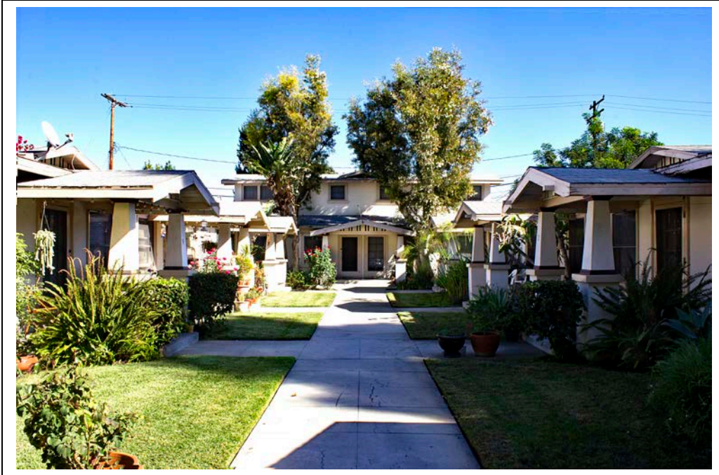
Figure 12: 2012 photo of Pomona Court, looking east inside entrance on Pomona Avenue Source: Fullerton Public Library, Local History Room
