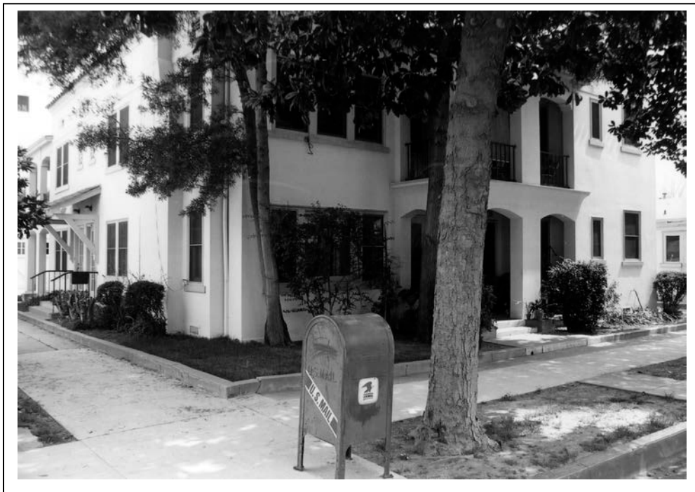
Figure 11: 1978 photo of Pomona Apartments, looking southeast from Pomona Avenue Source: Fullerton Public Library, Local History Room
